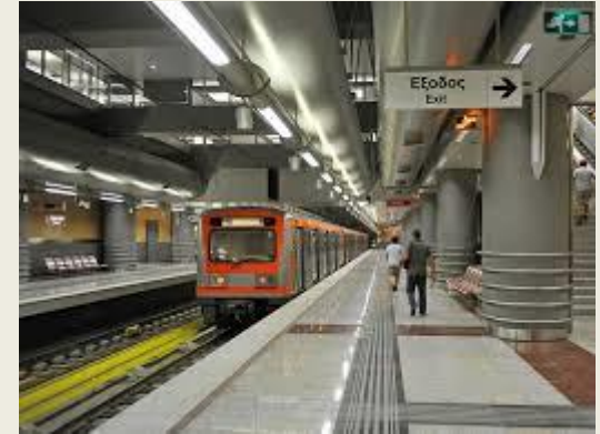
Athens Metro - Airport station
